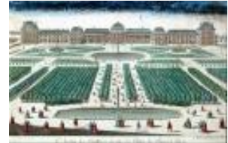
A view of the Tuilleries gardens in the 17 th century
